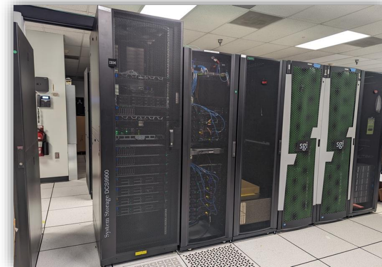
Explore Cloud Control Plane – Building 28
